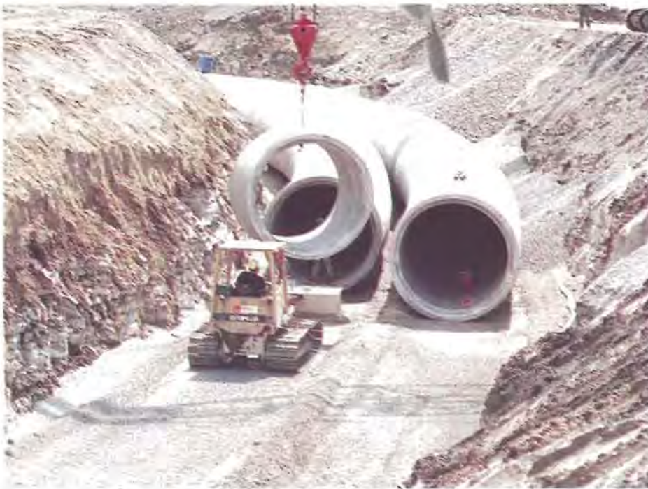
Installation of large-diameter concrete pipe
